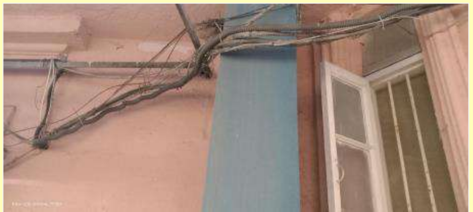
Exposed wirings in entire campus
