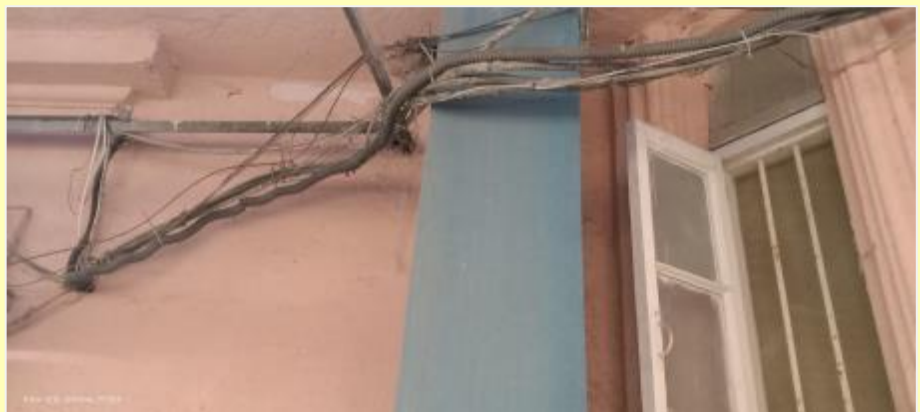
Exposed wirings in entire campus
